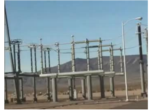
Lugo SWR: Electrical arc from power lines, by Neil Brady, 2013. Retrieved from www.youtube.com
